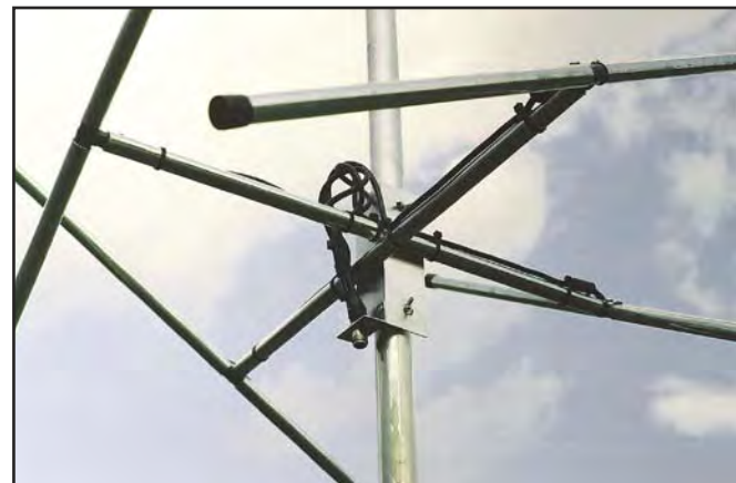
Figure 3 — View of cross booms mounted to mast.
