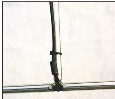
Figure 2 — Close-up of dipole electrical connections.
